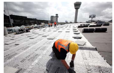
Especially for the Schiphol project ZinCo delivered the drainage element Fixodrain® XD 20 equipped with an additional protective rubber mat attached on the underside.
