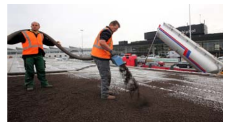
The System Substrate "Sedum Carpet" was brought up to the roof and distributed evenly by means of silos.
