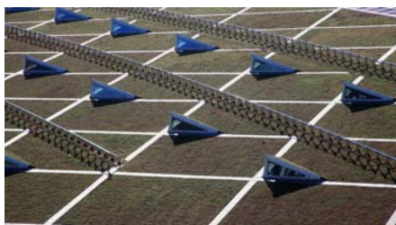
An immediate green coverage was achieved by applying pre-cultivated vegetation mats on the roof surface.
