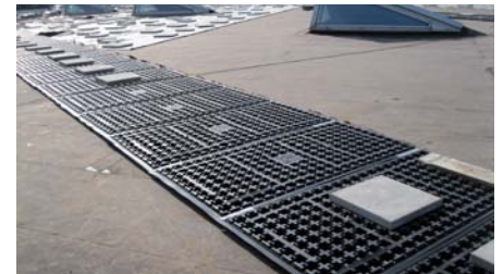
The Solar Bases® SB 200 allow for the installation of the solar modules, kept in place only by the weight of the green roof substrate itself.
